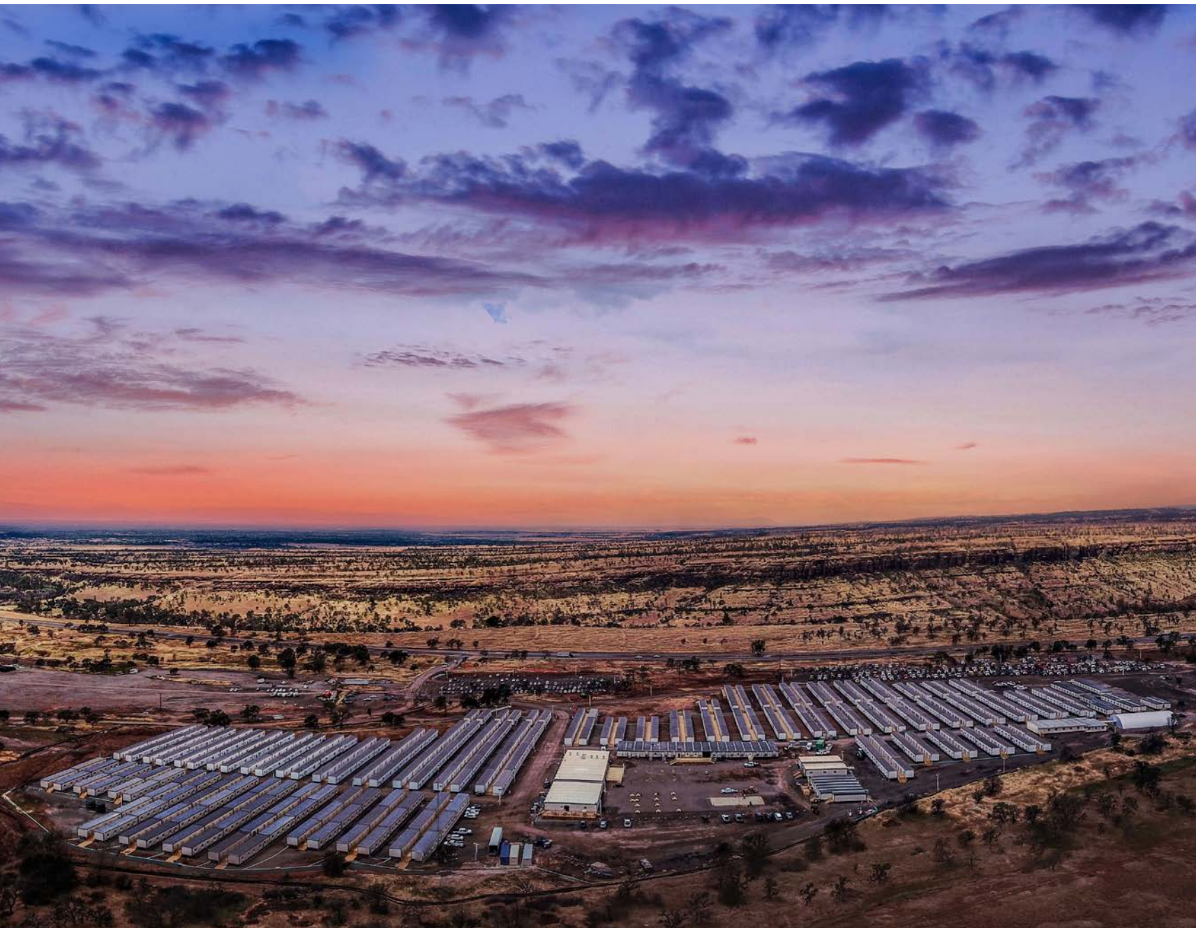
Our modular solutions can be rapidly deployed to respond to natural disasters and emergencies. The Tuscan Ridge Lodge in Butte County, California, was built to house 1,500 men and women supporting critical clean-up and restoration efforts after the wildfire in northern California.
