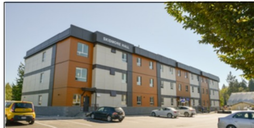
130-STUDENT DORMITORY Langley, Canada
