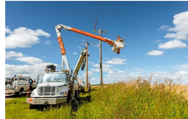
ELECTRICITY DISTRIBUTION $2.7B Rate Base
