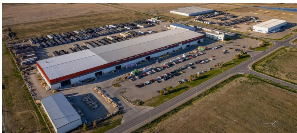
Triple M's 230,000 square foot manufacturing facility, Lethbridge, Alberta, Canada
