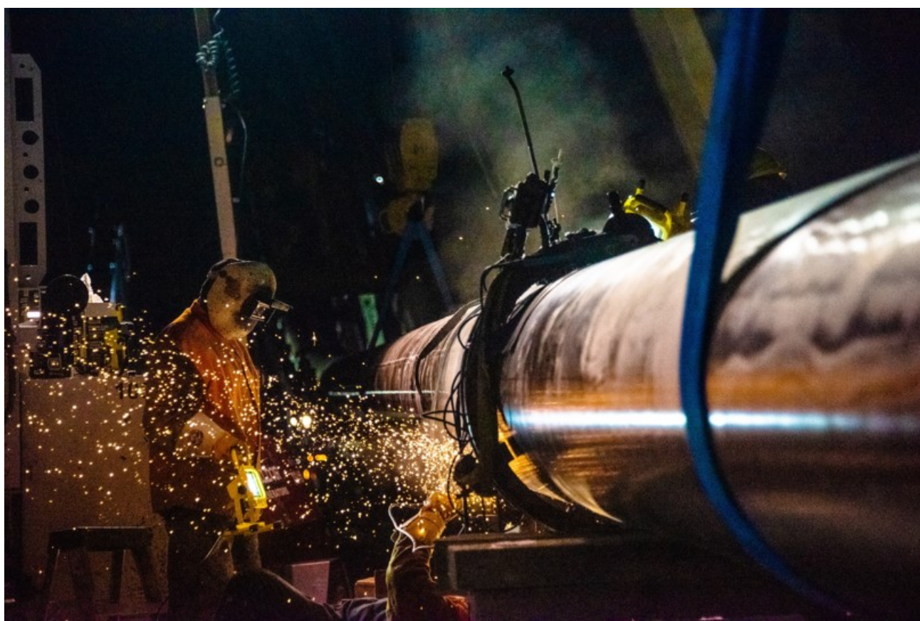
Pembina-Keephills transmission pipeline construction, near Wabamun Lake, Alberta
