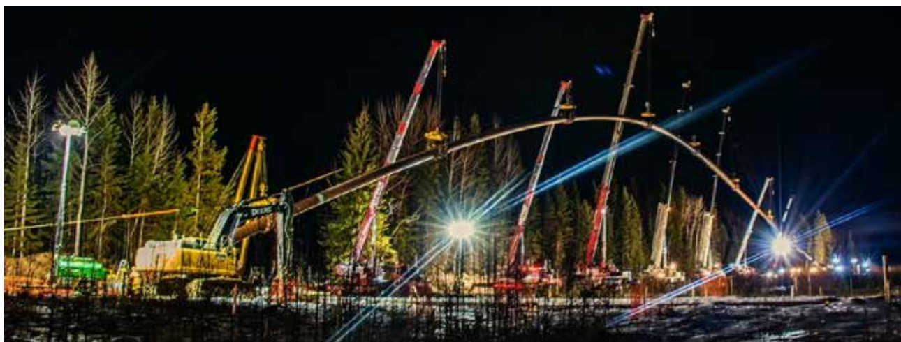
Pembina-Keephills transmission pipeline construction, near Wabamun Lake, Alberta
