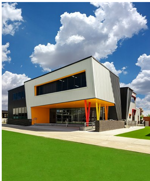
Permanent modular classroom, Victoria, Australia
