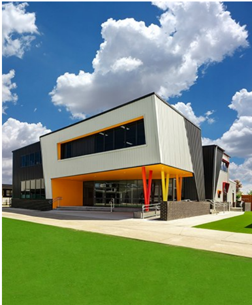
Permanent modular classroom, Victoria, Australia
