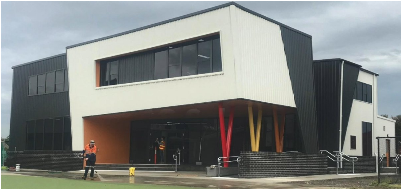
Permanent Modular classroom in the state of Victoria, Australia
