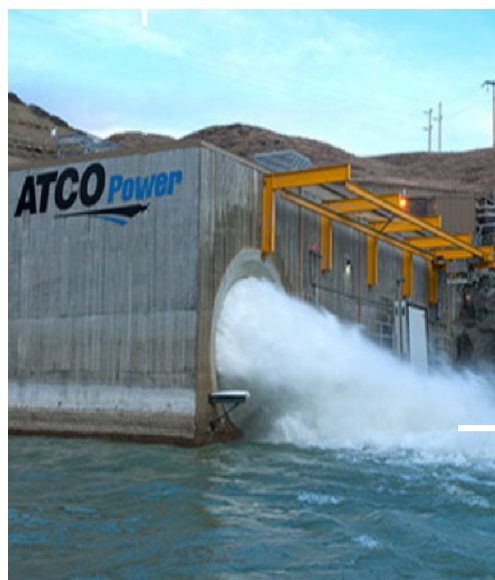
Oldman River Hydroelectric Plant
