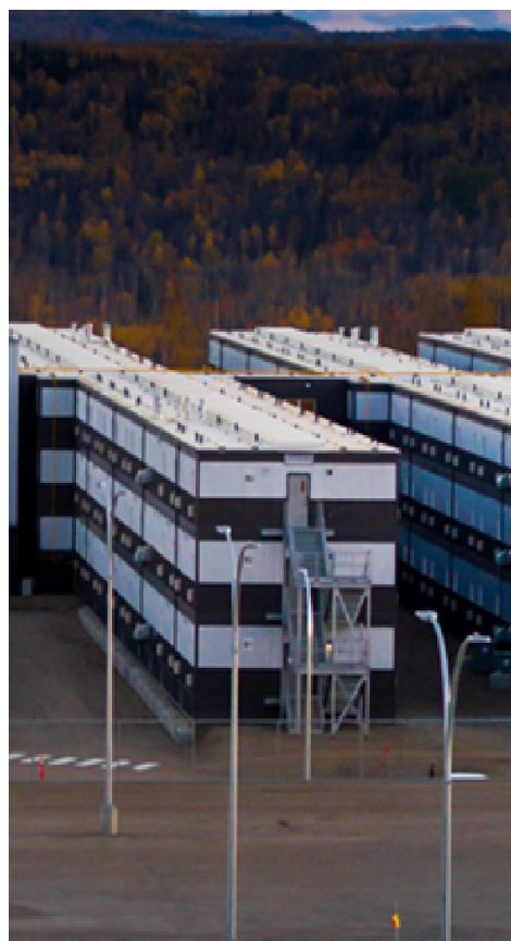
Site C Workforce Housing Camp
