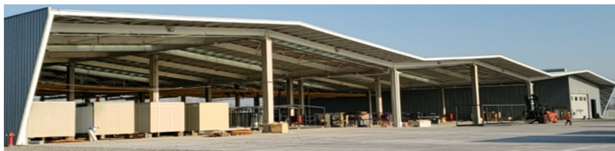
Chile Modular Structures Manufacturing Facility
