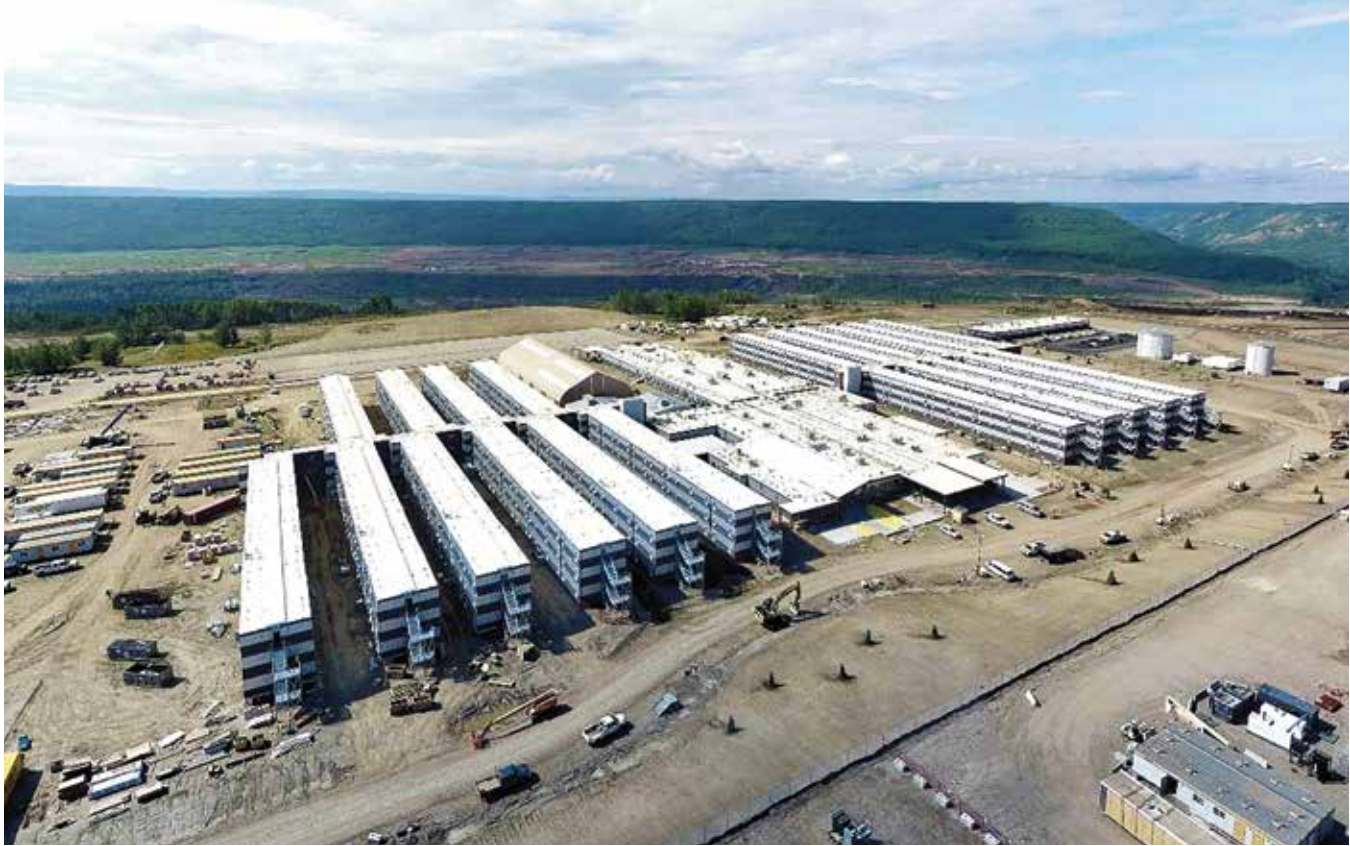
The 650,000 sq. ft. Site C Workforce Housing Facility was one of the largest construction projects in ATCO's history.
