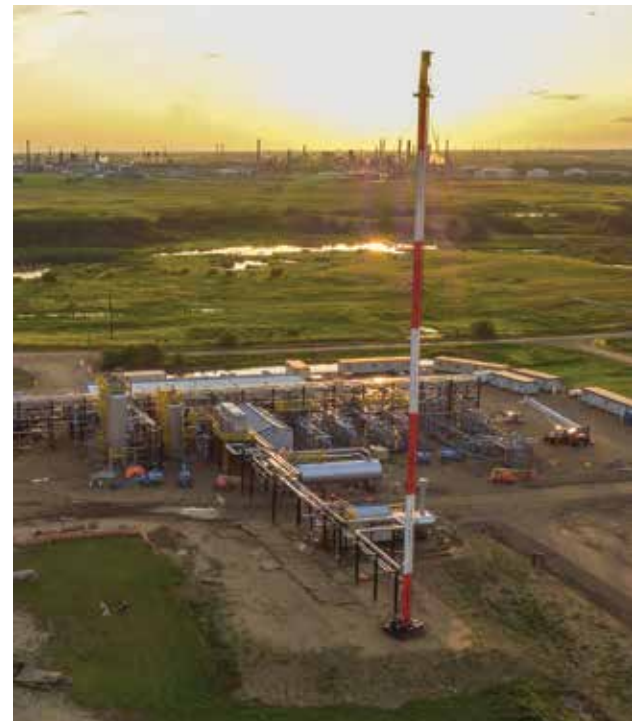
Our salt cavern facility at the ATCO Heartland Energy Centre allows us to leverage our industrial water infrastructure in the area to wash two caverns simultaneously which shortens development time. The central location also provides our customers with transportation options to solve the logistical challenges of moving product to market or securing it to avoid processing interruptions.
