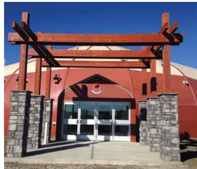
In 2016, we completed construction on a 39,000 sq. ft. Multi-Purpose Centre for the Piikani Nation.
