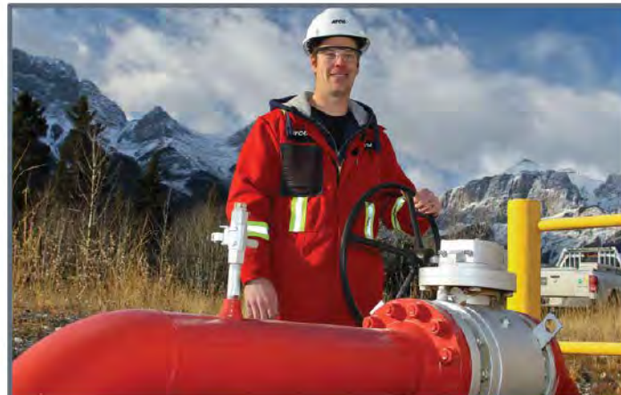
NATURAL GAS TRANSMISSION
